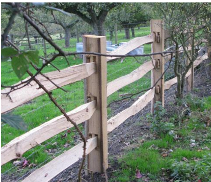
Appendix 1: Example cleft chestnut post and rail with stock netting
